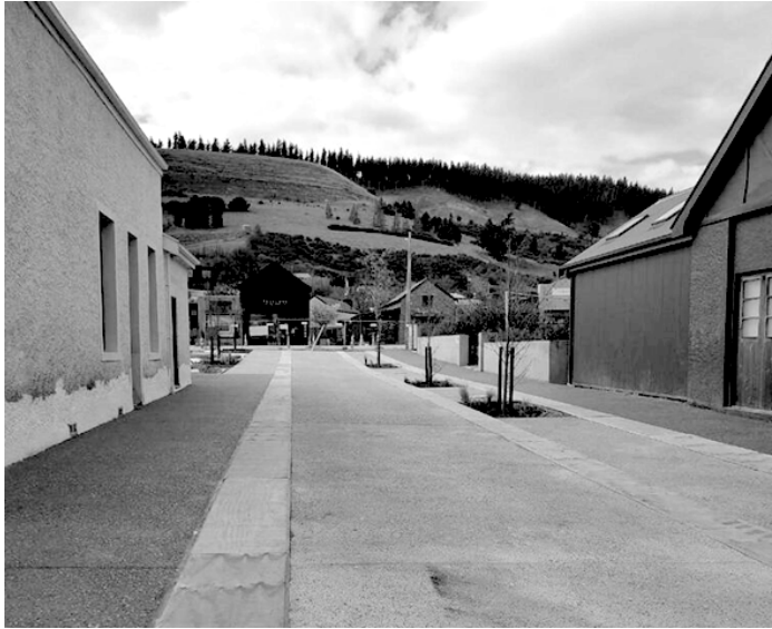
Early miners and townspeople would find it hard to believe that this is Clyde. Work began on upgrading the centre of the historic precinct in June and the result, says the Dunstan Times , does not disappoint. The pavers will be installed under the wooden strips once they arrive.
